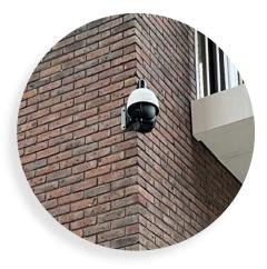
The CCTV system comprises 2nr 64ch NVRs linked to 119 IP cameras through POE layer 3 fibre switches. It features 8 PTZ cameras with configured patrols and offers remote access via both LAN and WAN connections.
